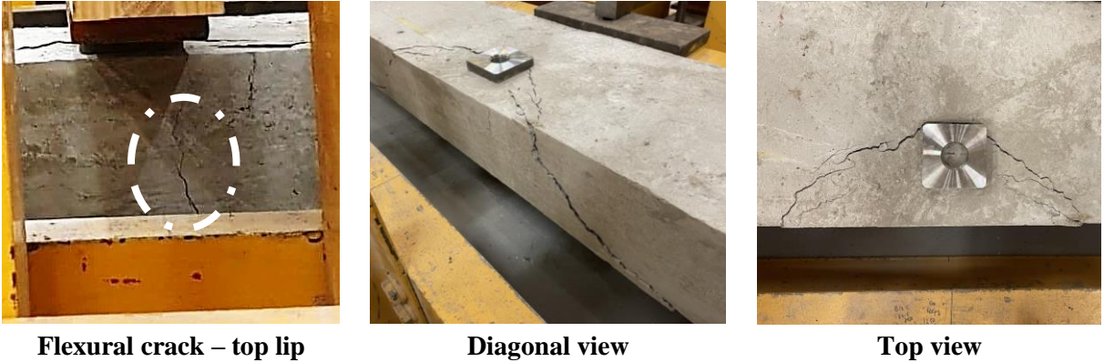
Figure 21. Test 3 observed failure
