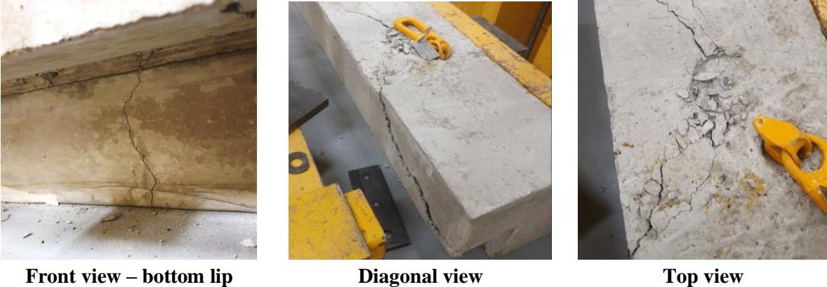
Figure 23. Test 4 observed failure
