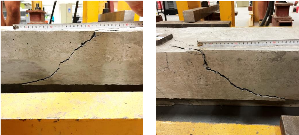
Figure 28. Measured front face of shear failure plane for test 3
