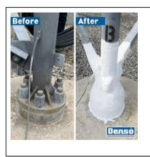
An example of a corrosion protection system that may be specified is the Denso SteelGard 400 (Butyl-based adhesive):
